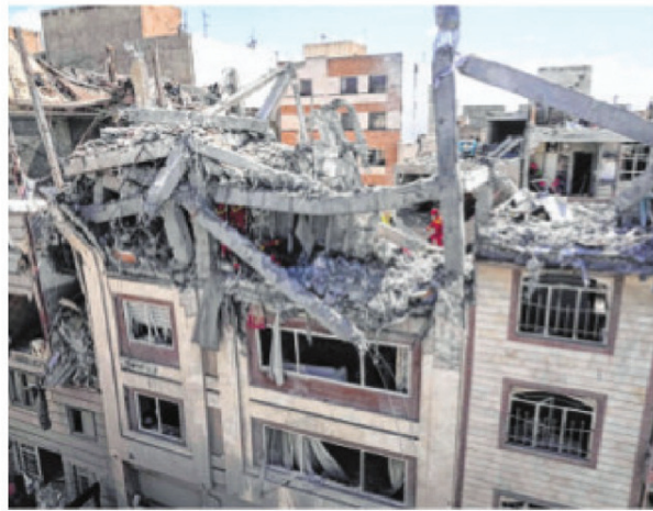
A damaged residential building in Tehran. —AP
